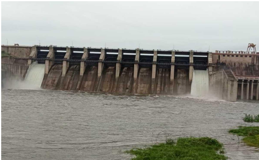
Figure 1. Yeldari Dam Parbhani district, Maharashtra.
